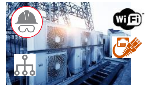
Air Conditioning Monitoring and Control for Hotels
